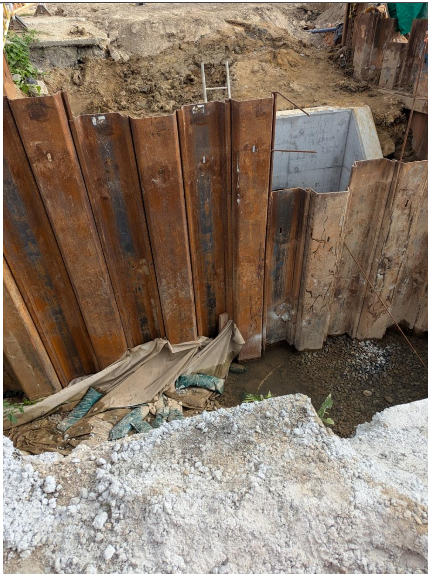
Photo 4 (Taken at CEDD Construction site on 26 May 2026)
