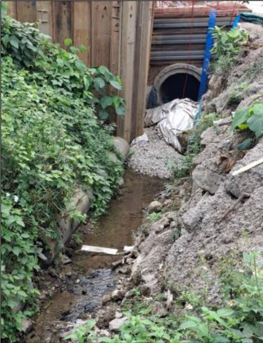
Photo 2a (Provided by CEDD, taken on 8 Apr 2026)
