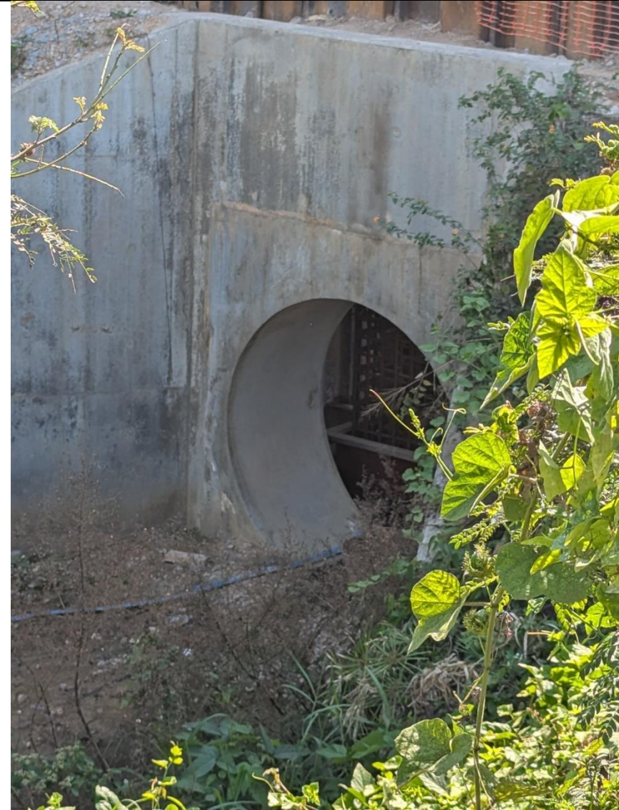
Photo 5b (Taken at Eastern portorm of HSKEPP on 13 Mar 2026)
