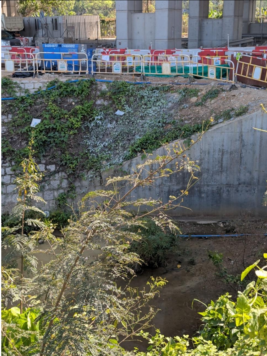
Photo 5a (Taken at Eastern portorm of HSKEPP on 13 Mar 2026)
