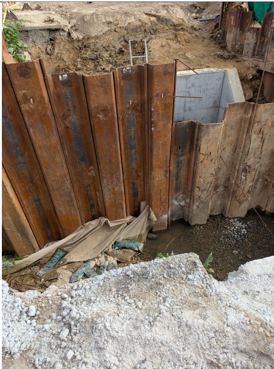
Photo 4 (Taken at CEDD Construction site on 26 May 2026)
