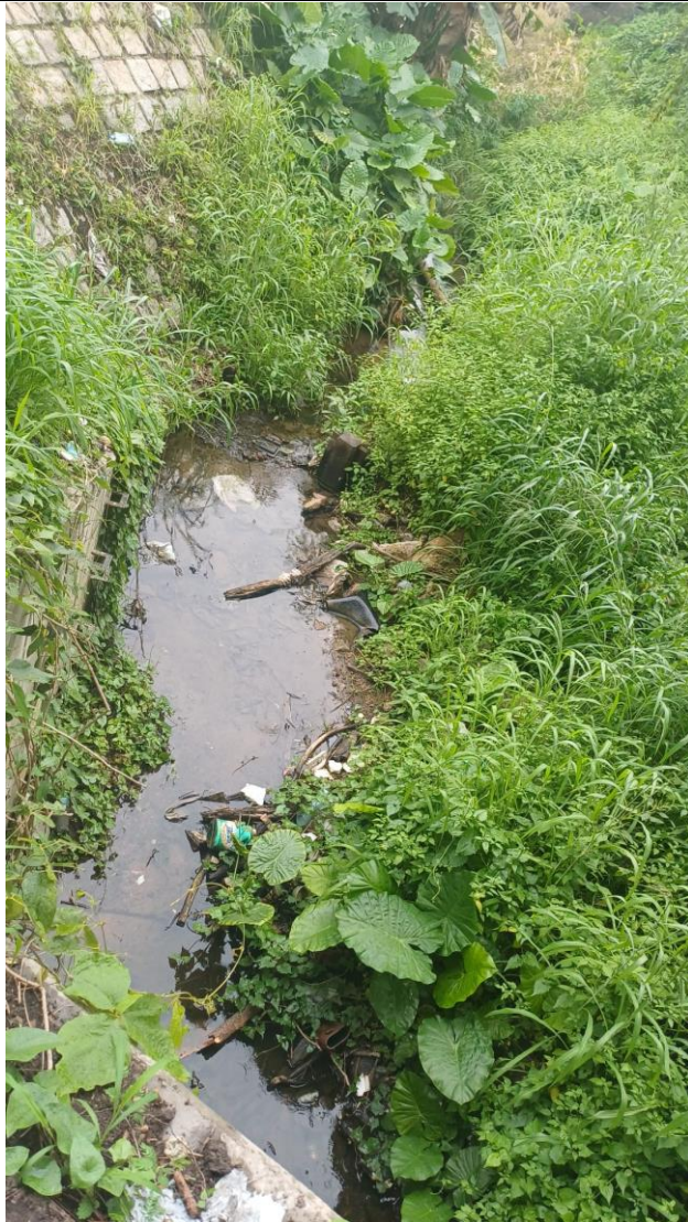
Photo 1a (Taken at C1 Station on 04 May 2026)
