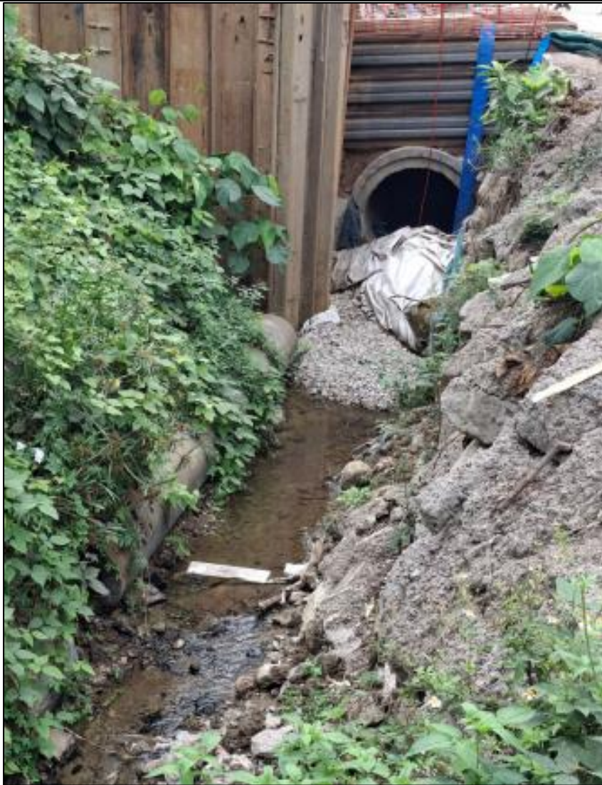
Photo 2a (Provided by CEDD, taken on 8 Apr 2026)
